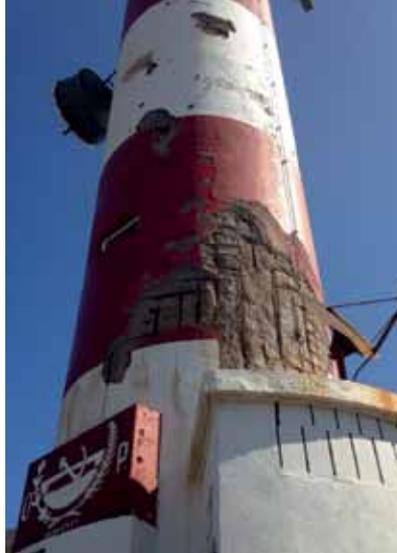
thixotropic mortar MAPEGROUT T40, which is easy to apply in thick layers on vertical surfaces without using formwork, mixed with MAPECURE SRA 25 (this product has now been replaced in Spain with MAPECURE SRA). On some of the smaller areas, on the other hand, PLANITOP SMOOTH & REPAIR fibre-reinforced, thixotropic cementitious mortar was applied.
