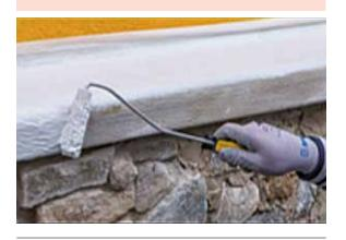
Two-component, CEMENT-FREE, LIME and Eco-Pozzolan based coating for **waterproofing** and **protecting** construction features, including those of historical and artistic interest.
