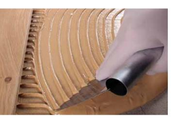
One-component, solvent-free, ready-mixed, elastic polyurethane adhesive with very low emission of volatile organic compounds (EMICODE EC1 R Plus) for all types of pre-finished ply parquet and traditional, solid tongue and grooved wooden planks
