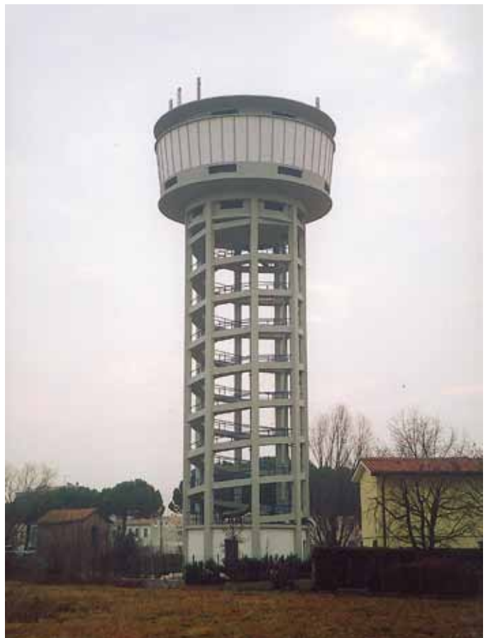
Suspended water tank - Rovigo - Italy
