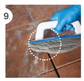
Grout the gaps and seal all the joints and fillets
