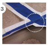
Apply **Mapeband** tape along the control joints and the fillets between floors and walls. The ends must be bonded together with **Adesilex LP**
