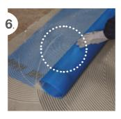
Waterproof the area by applying the first coat of **Mapelastic Turbo** and apply **Mapenet 150** or **Mapetex Sel** over the waterproofing product
