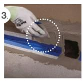
Apply **Mapeband** tape along the check joints and the fillets between floors and walls. The ends must be bonded together with **Adesilex LP**
