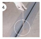
Bond **Mapeband TPE** with **Adesilex PG4** adhesive on structural joints and broadcast the surface with quartz sand. The ends must be bonded together with **Adesilex LP** or hot-welded
