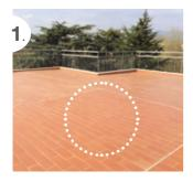
Check that the existing coating material is well bonded. Prepare all surfaces by sanding or cleaning them thoroughly with caustic soda; rinse the surfaces
