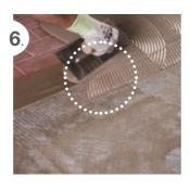
Waterproof the area by applying a first coat of **Mapelastic Turbo** and apply **Mapenet 150** or **Mapetex Sel** over the waterproofing product
