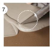
When the first coat is dry, apply the second coat of **Mapelastic Turbo**
