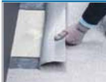
Double-sided adhesive band for installing removable resilient and textile floor coverings.
