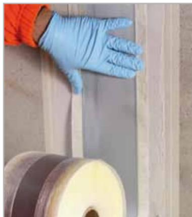
Fig. 7.48c - Positioning MAPEBAND TPE
