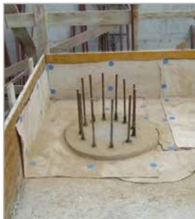
Fig. 7.20 - MAPEPROOF cut to shape around the head of a pile
