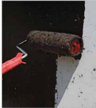
Fig. 7.51 – Using a roller to apply PLASTIMUL PRIMER
