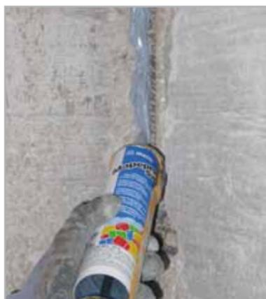
Fig. 8.1b - Extrusion of MAPEPROOF SWELL
