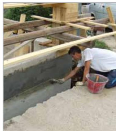
Fig. 7.47 – Application of MAPELASTIC FOUNDATION with a brush on the upper part of a wall before applying MAPEPROOF
