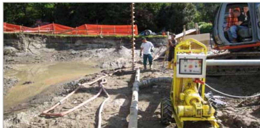
Fig. 3.6 – Drilling operations to insert wellpoints
