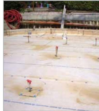
Fig. 7.27 – An overall view of the waterproofing layer on the head of a series of piles
