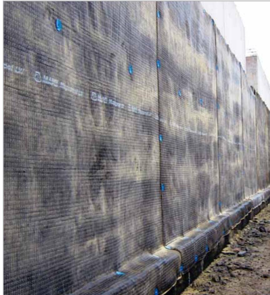
Fig. 5.3 – An example of MAPEPROOF applied after casting
