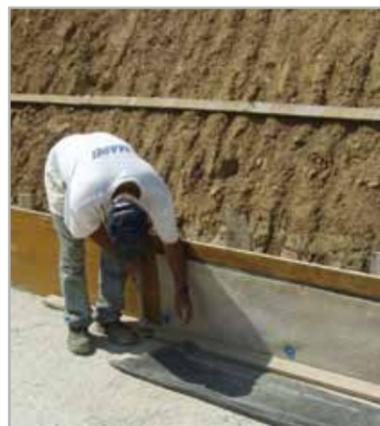
Fig. 7.10 – Nailing MAPEPROOF to wooden formwork
