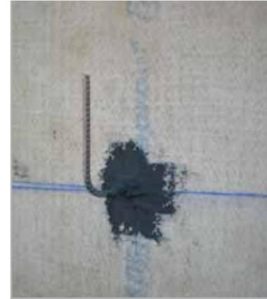
Fig. 7.69 - Grouting metallic connectors with MAPEPROOF MASTIC
