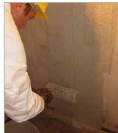
Fig. 8.8e – Application of **MAPELASTIC FOUNDATION**
