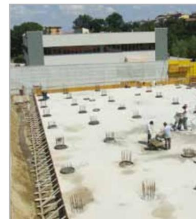
Fig. 7.18 - An overall view of a series of piles during the rebuilding of the heads
