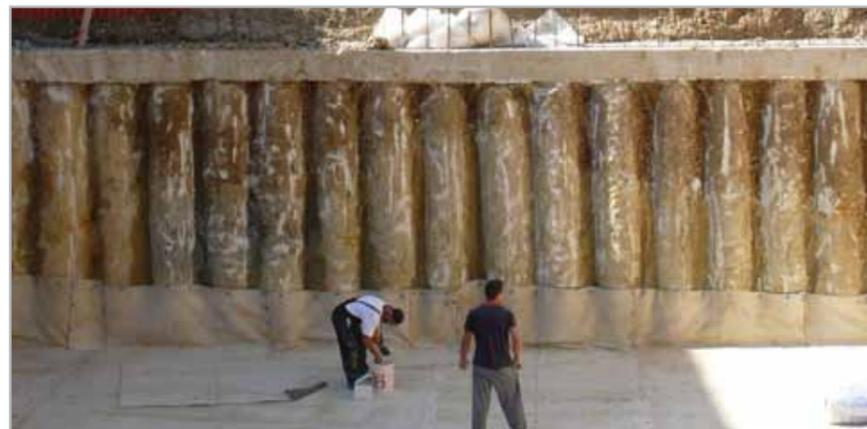
Fig. 7.32 – MAPEPROOF applied directly on a pile bulkhead
