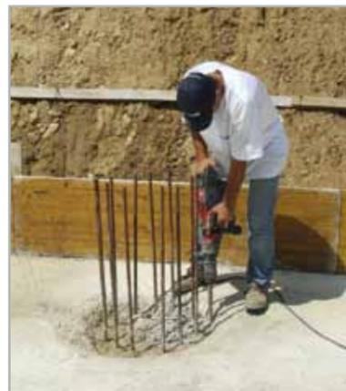
Fig. 7.15 - Cropping the head of a pile
