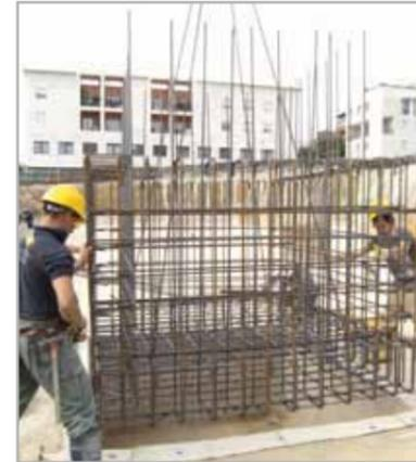
Fig. 7.5c – Positioning the steel reinforcement
