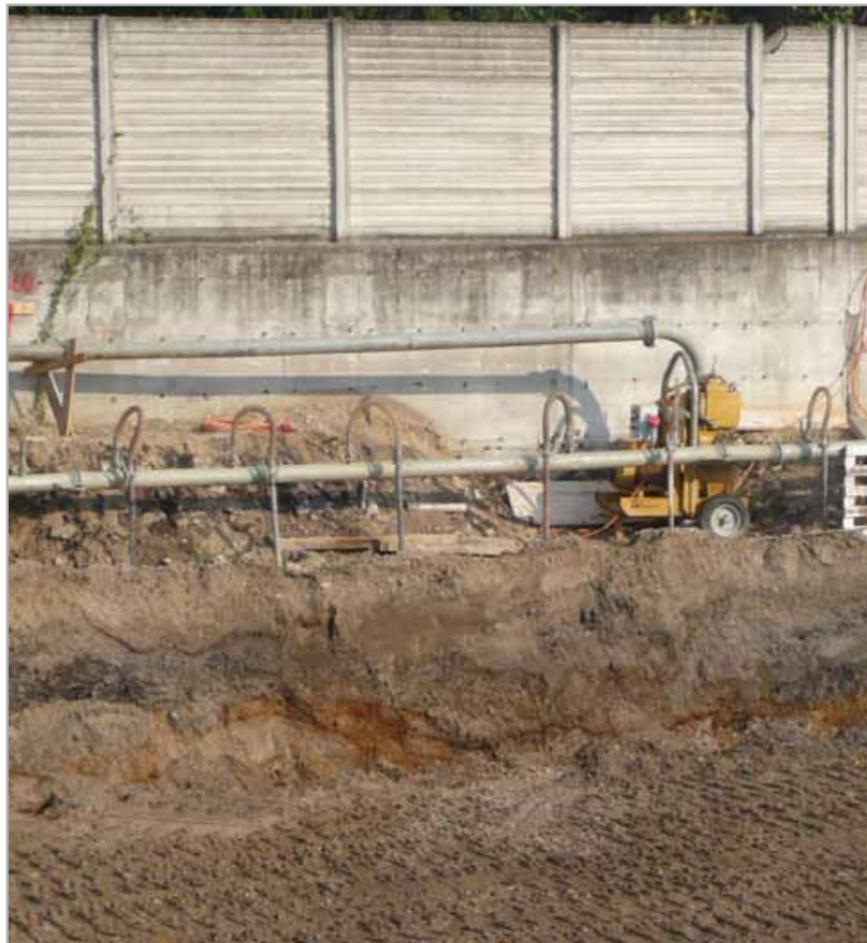
Fig. 3.7 – Centrifugal pump used in a wellpoint system
