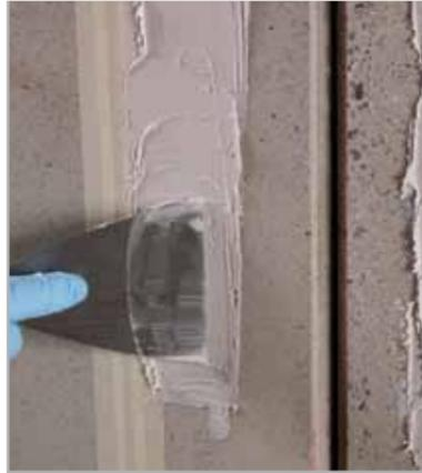
Fig. 7.48b - Spreading on ADESILEX PG4 with a trowel
