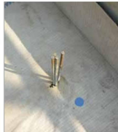
Fig. 7.24 - MAPEPROOF with the steel reinforcement of a pile passing through it
