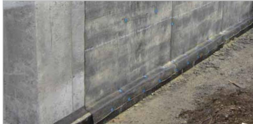
Fig. 7.45A – Nailing MAPEPROOF to the substrate after casting
