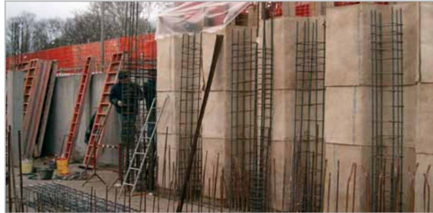
Fig. 7.31 – MAPEPROOF applied directly on sheetpiling
