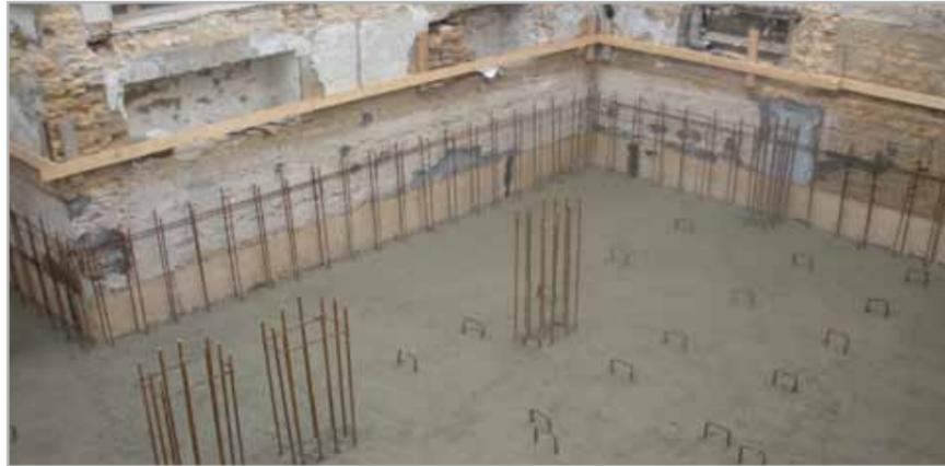
Fig. 8.5c - Reinforced concrete floor slab cast on the MAPEPROOF at a thickness calculated to withstand hydraulic lift from the groundwater
