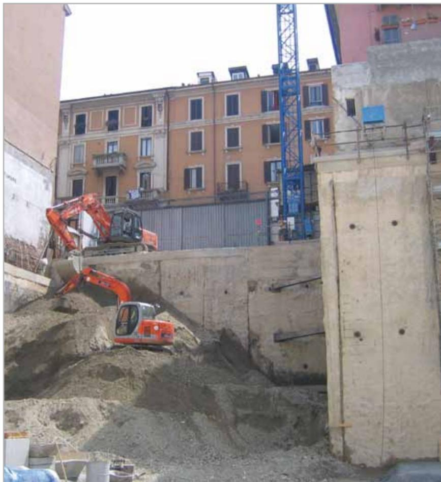
Fig. 1.1 – Phases of an excavation for construction work carried out below ground level in a built-up area
