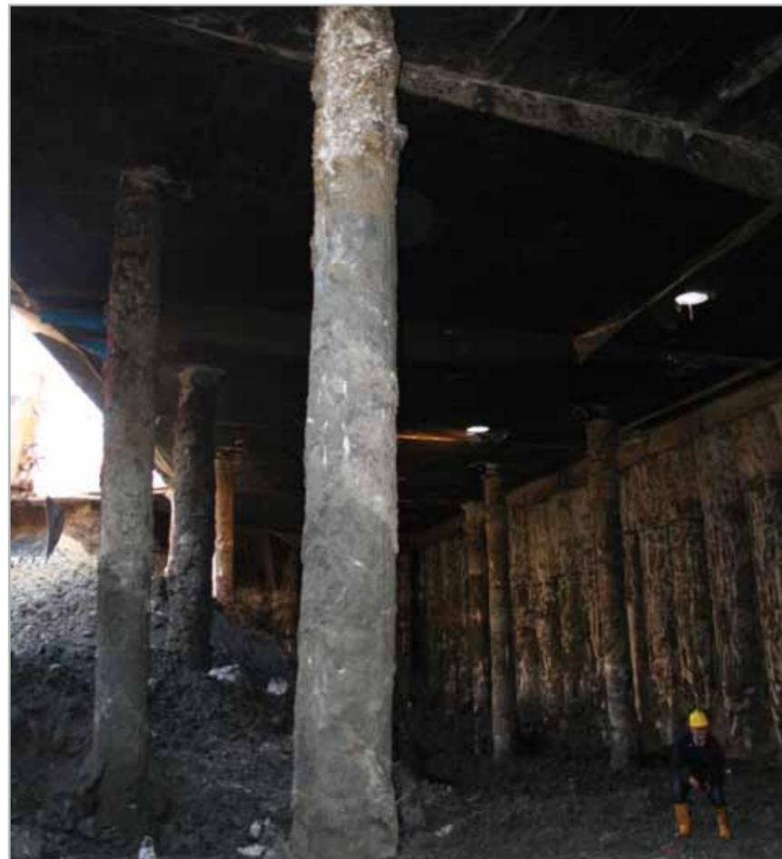
Fig. 4.5 – Example of a Top-Down construction. Excavation work carried out under the reinforced concrete foundation pad cast before excavating
