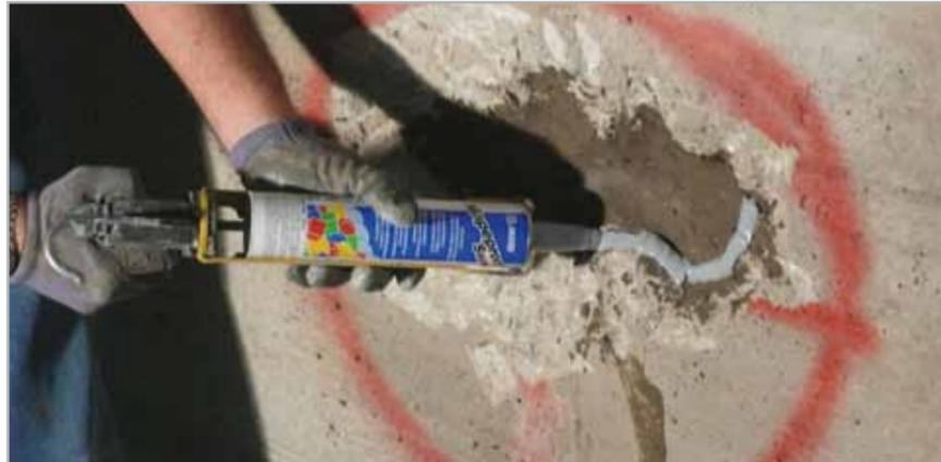
Fig. 8.3 – Extrusion of MAPEPROOF SWELL on a zone damaged by seeping water blocked beforehand with LAMPOSILEX
