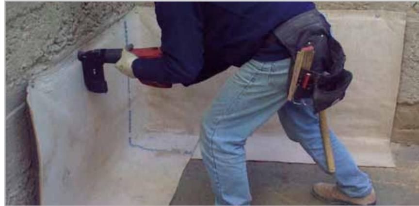
Fig. 8.5a – One of the phases of lining the inside of a room with **MAPEPROOF** on the horizontal and vertical surfaces: application of **MAPEPROOF** on the lower part of the vertical walls with the sheet hemmed over onto the lean concrete
