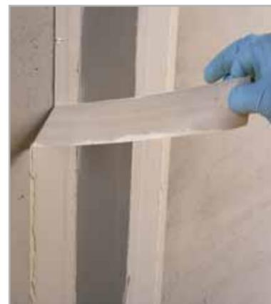
Fig. 7.48e – Before reticulation of ADESILEX PG4, sprinkle quartz sand on the surface and remove the masking tape
