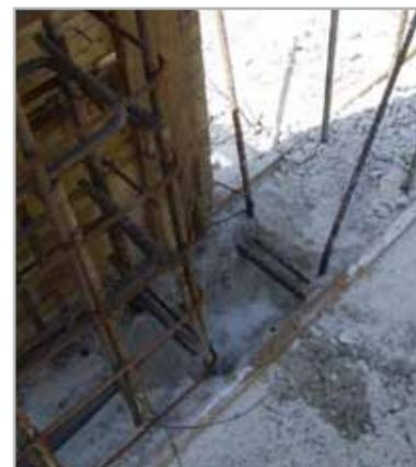
Fig. 7.56b – Demolition to a depth of 15 cm from the upper part of the foundation pad
