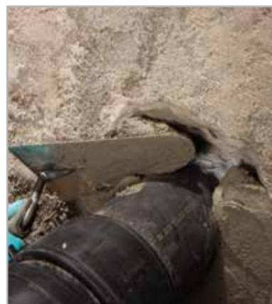
Fig. 8.2 - Sealing a pipe passing through the surface by extruding MAPEPROOF SWELL and then confining the pipe with MAPEGROUT BM
