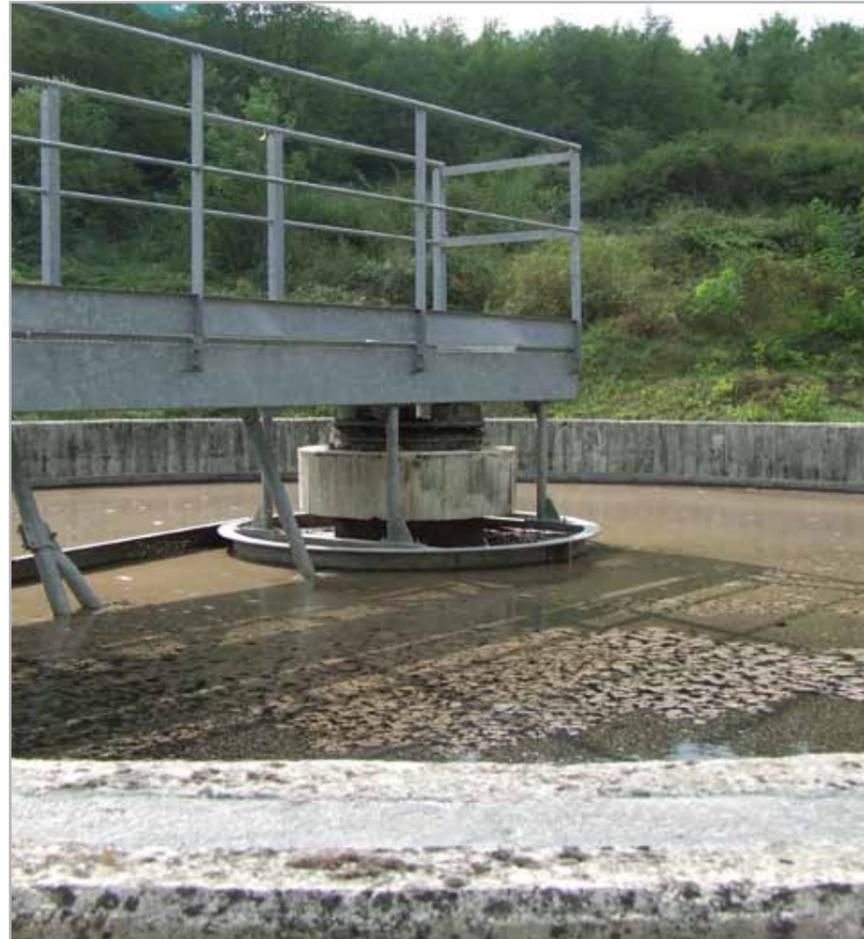
Fig. 7.64 – Sedimentation tank in an advanced state of deterioration
