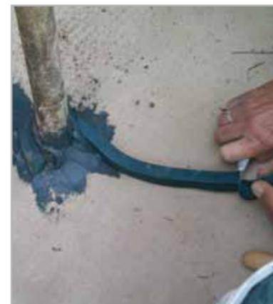
Fig. 7.60c – Laying IDROSTOP B25
