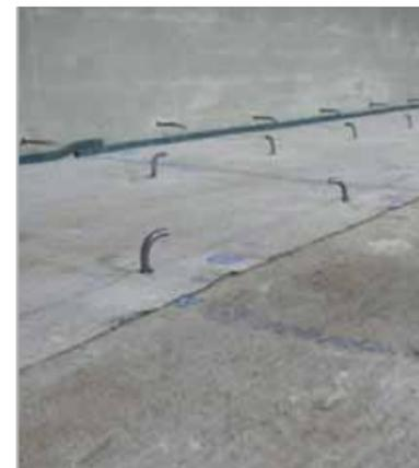
Fig. 8.6d - Metal connectors are required to make the new structure part of the existing one
