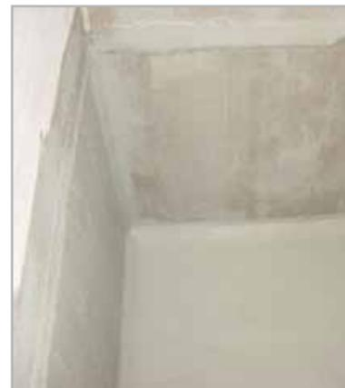
Fig. 8.8e – Vertical walls and horizontal surfaces waterproofed with **MAPELASTIC FOUNDATION**
