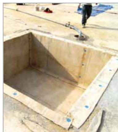
Fig. 7.5b – Lift well lined with MAPEPROOF
