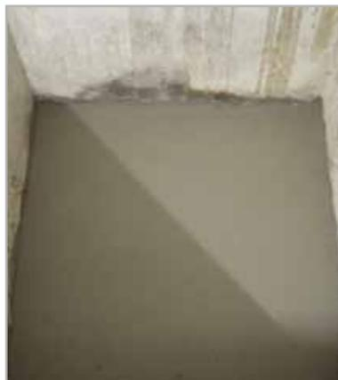
Fig. 8.8b – Screed made from sand, cement and **IDROSILEX**
