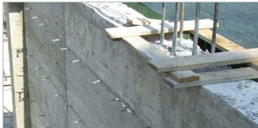
Fig. 7.43 – The blades of the formwork sticking through a reinforced concrete wall before being removed
