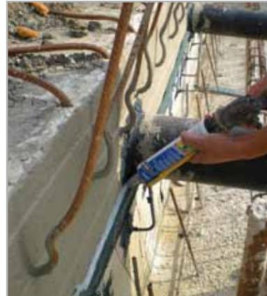
Fig. 7.72 – Extrusion of MAPEPROOF SWELL onto IDROSTOP B25 in the fillet joint between MAPELASTIC FOUNDATION and MAPEPROOF
