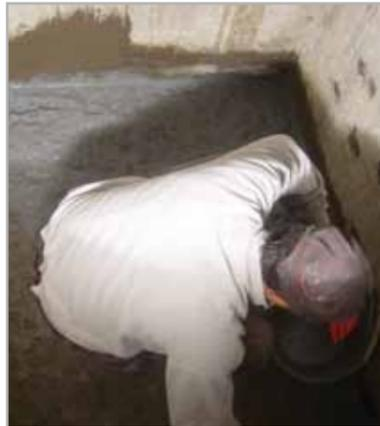
Fig. 8.8a – One of the phases of the installation of waterproof coating with water-repellent **IDROSILEX** mortar on the horizontal surface and **MAPELASTIC FOUNDATION** on the vertical and horizontal surfaces: spreading on bonding slurry
