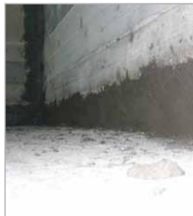
Fig. 8.1e - A sealed, repaired construction joint
