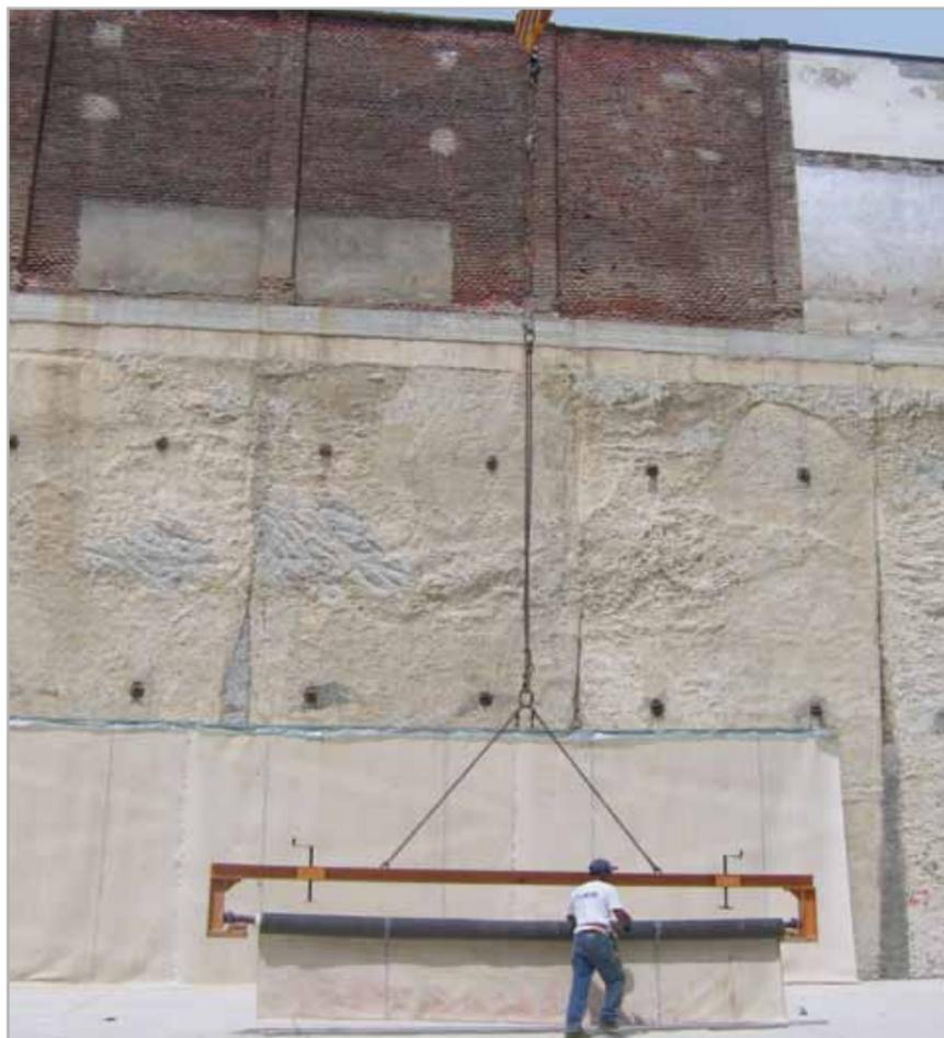
Fig. 7.37 - Laying MAPEPROOF against a diaphragm
