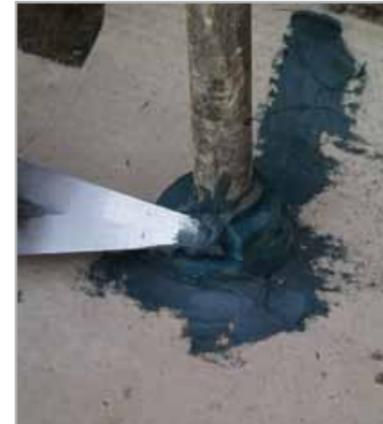
Fig. 7.60e - Further grouting with MAPEPROOF MASTIC
