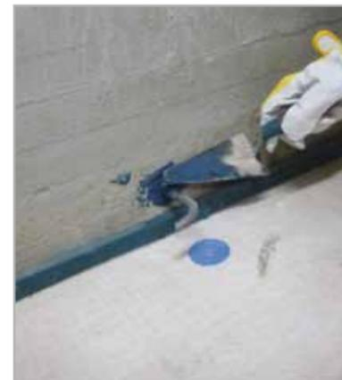
Fig. 8.6f - Grouting the metal connectors with MAPEPROOF MASTIC
