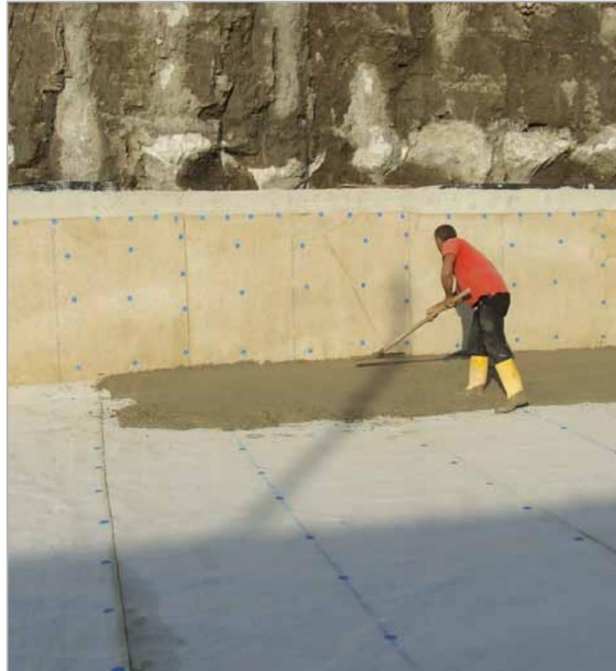
Fig. 7.9 – One of the phases of casting the protective layer of concrete on MAPEPROOF, using concrete with the same Rck as that of the foundation pad
