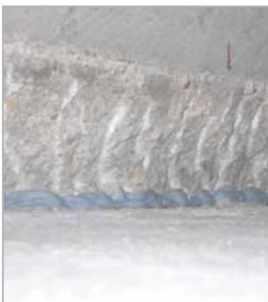
Fig. 8.1c - Construction joint sealed with MAPEPROOF SWELL
