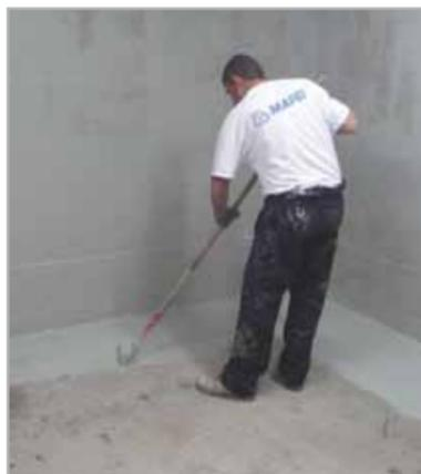
Fig. 8.6a - One of the phases of relining the inside of a room with MAPELASTIC FOUNDATION on the vertical walls and MAPEPROOF on the horizontal surfaces: application of MAPELASTIC FOUNDATION on the vertical walls and on the new lean concrete at a width of at least 50 cm
