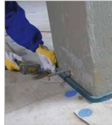
Fig. 8.6e - Lay IDROSTOP B25 in correspondence with the joints between MAPELASTIC FOUNDATION and MAPEPROOF
