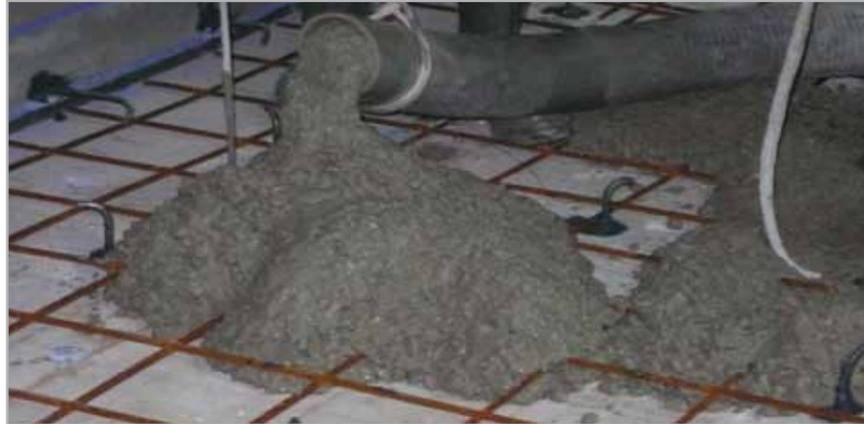
Fig. 8.6h - Casting of the reinforced concrete floor slab, calculated to withstand the hydraulic lift from the groundwater
