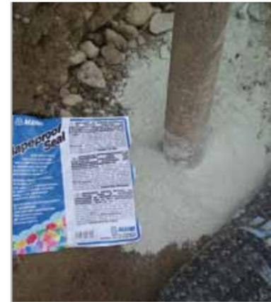
Fig. 7.60a – One of the phases of sealing a pipe which passes through the foundation pad: application of MAPEPROOF SEAL around the pipe
