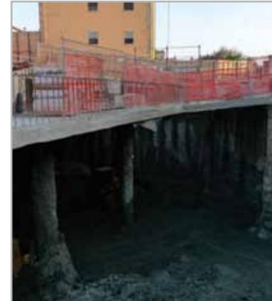
Fig. 7.73 - Excavation work carried out under the reinforced concrete foundation pad cast before excavating
