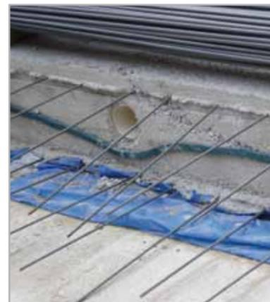
Fig. 7.29 – Sealing a construction joint on a foundation pad with IDROSTOP B25. The protective PE sheet on the strip of MAPEPROOF may be seen protruding from the foundation, which is then overlapped with the adjacent sheet laid before casting the next layer of concrete
