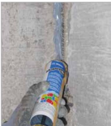
Fig. 8.1b - Extrusion of MAPEPROOF SWELL
