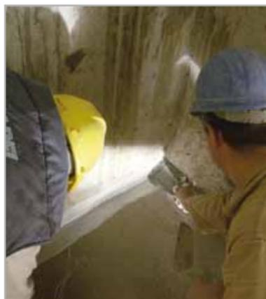
Fig. 8.8c – Application of **EPORIP** in the fillet joints between horizontal and vertical surfaces and between adjacent walls
