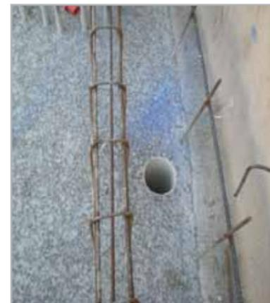
Fig. 7.75 – A hole left in the floor slab to pour concrete into the vertical walls
