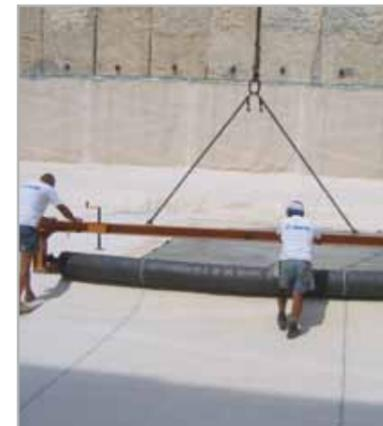
Fig. 7.12 – Laying MAPEPROOF using a metal lifting rig
