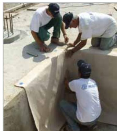
Fig. 7.5a – One of the phases of waterproofing and casting a lift well: application of MAPEPROOF on the side walls of the excavation
