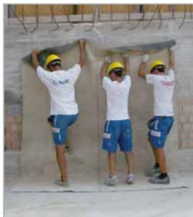
Fig. 7.68 - Bentonite sheet laid on the vertical surface and then hemmed over onto the horizontal surface
