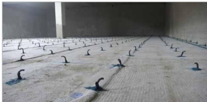
Fig. 8.6g - Metal connectors grouted before positioning the steel reinforcement for the new floor slab to be installed
