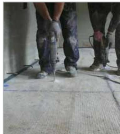
Fig. 8.6c - After laying MAPEPROOF on the lean concrete, make holes to insert the metal connectors
