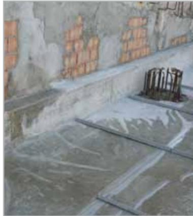
Fig. 7.66 - Application of a sheet of PE to form a floor slab with a regular inner side
