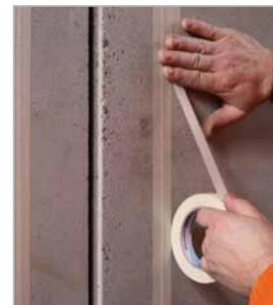
Fig. 7.48a – Phases of waterproofing an expansion joint subject to movements of up to 10 mm with MAPEBAND TPE: to avoid the epoxy adhesive leaving a rough edge, apply masking tape along the sides of the joint
