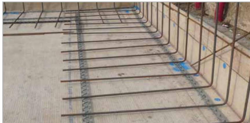
Fig. 7.13 – Metallic reinforcement positioned on MAPEPROOF and separated from the sheets with spacers
