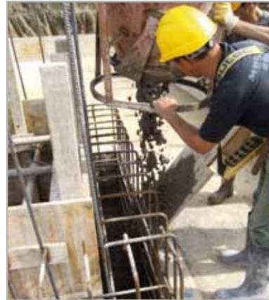
Fig. 7.5f – Casting vertical walls
