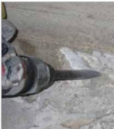
Fig. 8.1a - One of the phases of sealing a construction joint: mechanical demolition around a construction joint to a depth of approximately 6 cm
