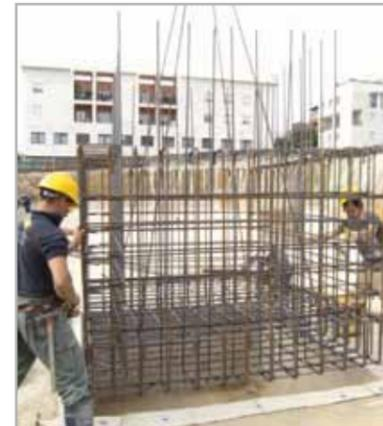
Fig. 7.5c – Positioning the steel reinforcement
