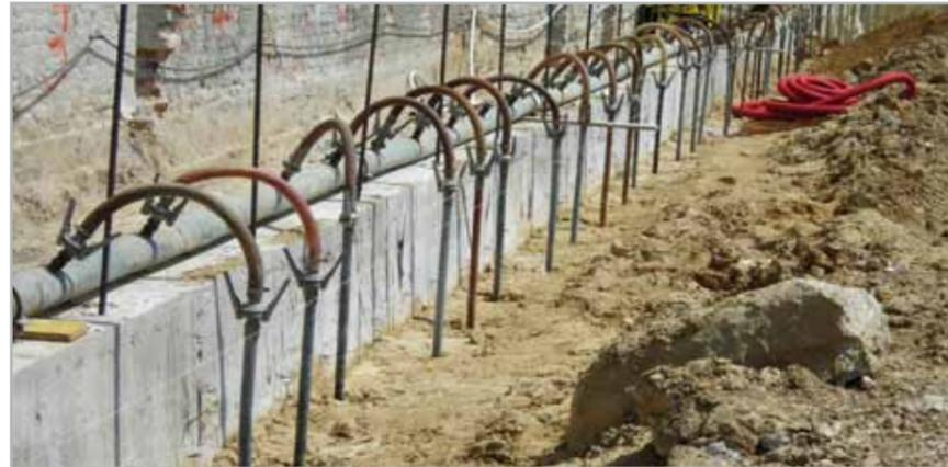
Fig. 3.4 – Flexible house used to connect wellpoints to an intake manifold
