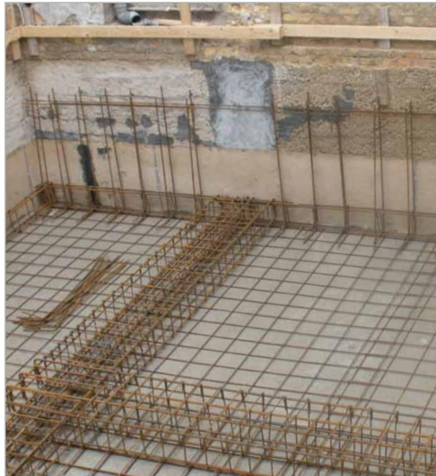
Fig. 8.5b – After laying the sheet on the horizontal surface, the steel reinforcement for casting the reinforced concrete floor slab and counter-wall is placed in position
