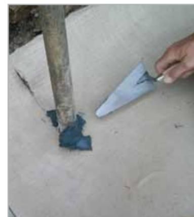
Fig. 7.60b – Application of MAPEPROOF MASTIC on the sheet
