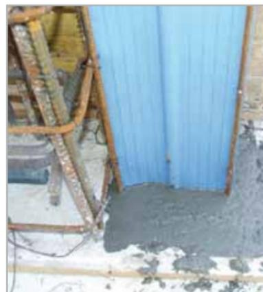
Fig. 7.56e – Repairing foundations with MAPEGROUT COLABILE
