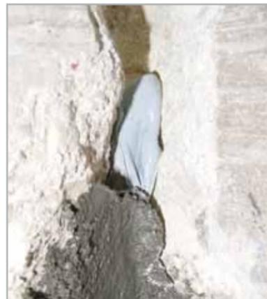
Fig. 8.1d - Confinement of MAPEPROOF SWELL by applying MAPEGROUT T40
