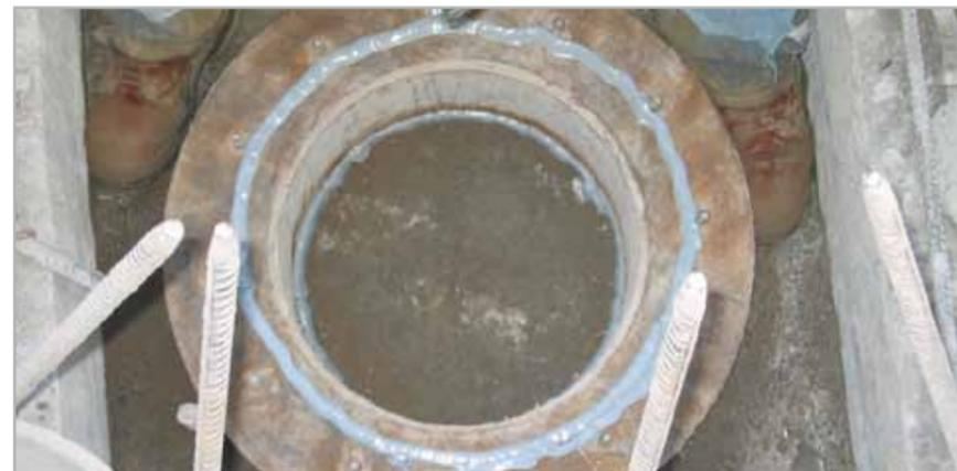
Fig. 7.61 - Extrusion of MAPEPROOF SWELL to seal the joint between a manhole cover and a well
