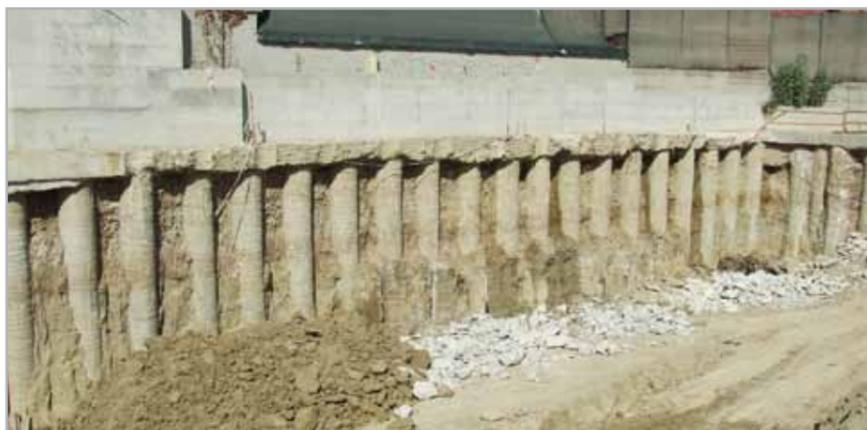
Fig. 4.3 – Stripped ground confined by bored piles
