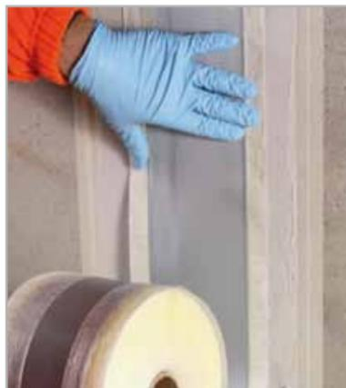
Fig. 7.48c – Positioning MAPEBAND TPE
