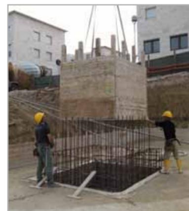
Fig. 7.5e – Positioning wooden formwork before sealing construction joints between a foundation pad and the walls using IDROSTOP B25
