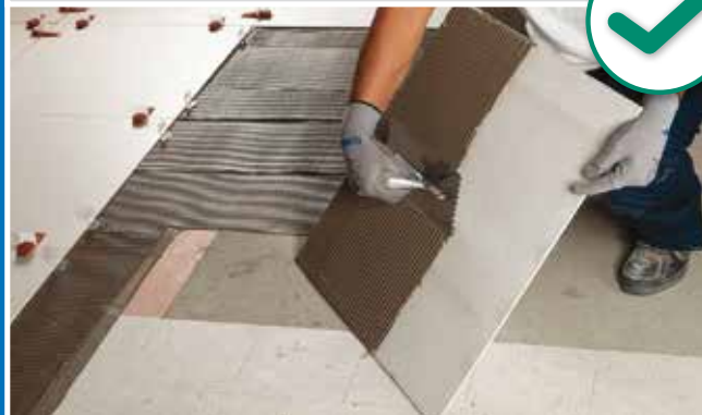
Posa conforme a UNI 11493
