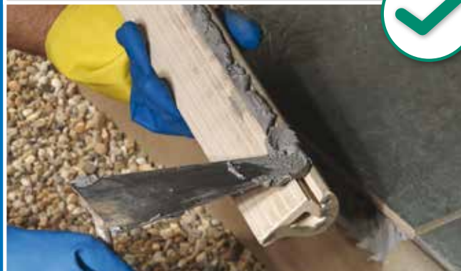
Posa conforme a UNI 11493
