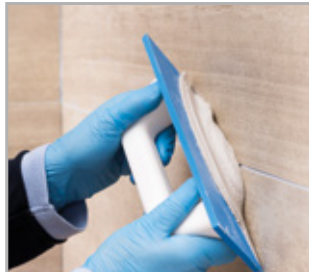
Grouting with Kerapoxy 4 LVT
