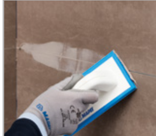
Grouting with Kerapoxy 4 LVT
