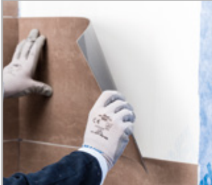
Installation of LVT on wall with Ultrabond Eco MS 4 LVT Wall
