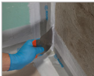
Waterproofing internal corners correctly by applying Mapeband PE120 and specially shaped pieces
