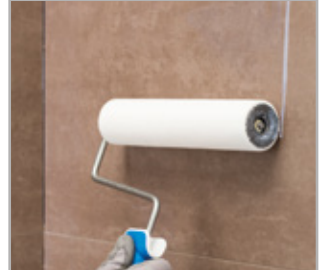
Application of Mapecoat 4 LVT
