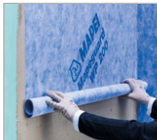
Application of Mapeguard WP 200
