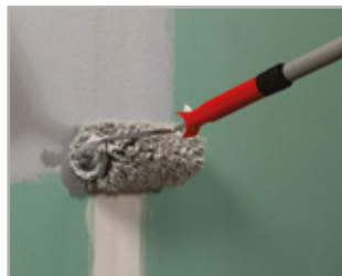
Spreading the first coat of Mapegum WPS
