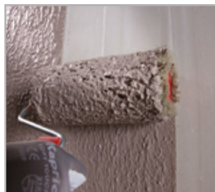
Spreading the first coat of Mapelastic Smart with a roller
