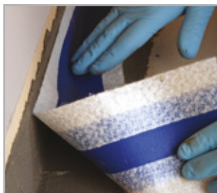
Applying Mapeband with Mapelastic Smart
