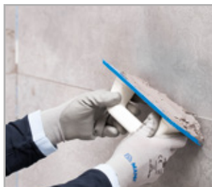
Grouting with Kerapoxy 4 LVT
