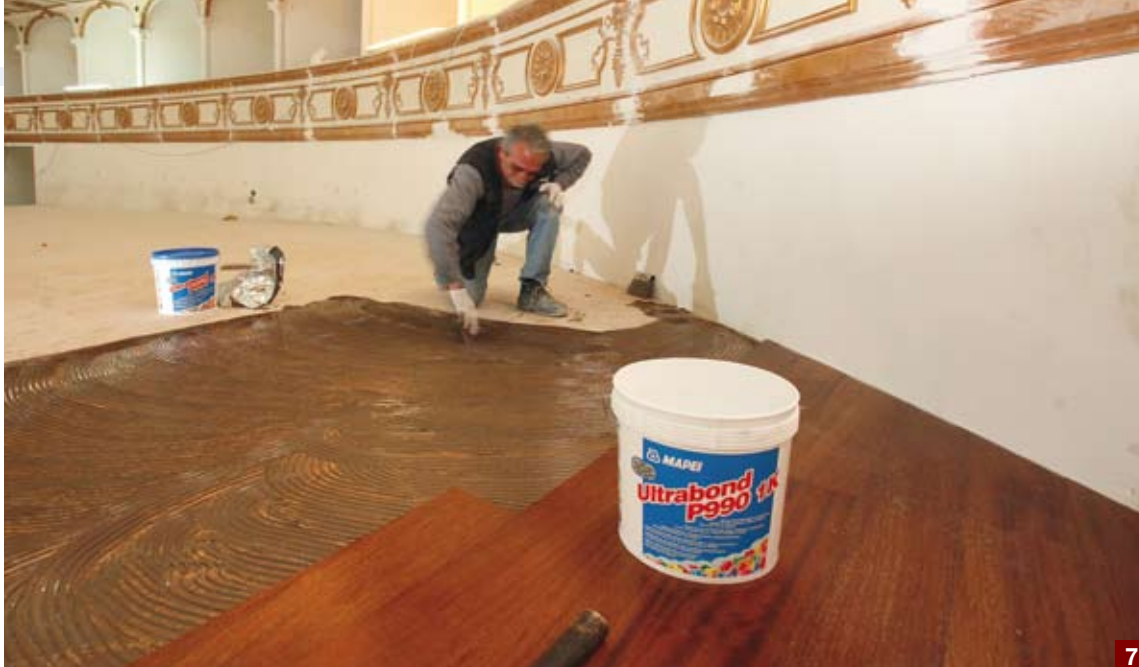
Photo 7. The pre-finished Iroko parquet in the stalls area was laid with ULTRABOND P990 1K.
