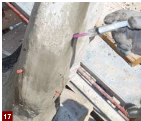
Photos 16, 17 and 18. The concrete statues, part of the pediment of the Petruzzelli Theatre, were renovated using MAPEFER, MAPEGROUT T40 and MAPEFINISH and consolidated with carbon fibre fabric from the MAPEWRAP range.
