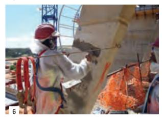
layers ranging from 25 mm to 30 mm. Some damaged areas also required the use of MAPEGROUT HI-FLOW (COLABILE) shrinkagecompensated fibre-reinforced grout.
