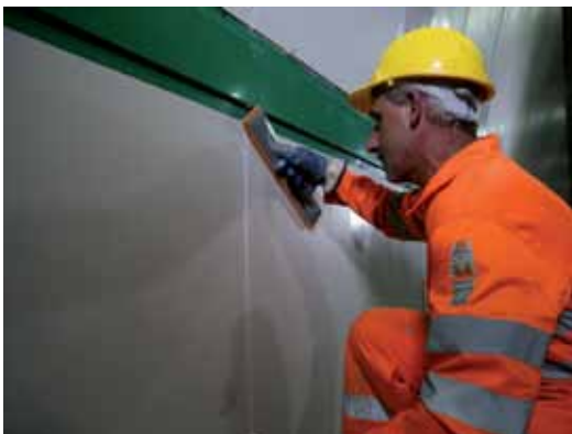
IN THESE PICTURES. Large-size ceramic tiles were bonded in the tunnel with KERAFLEX MAXI S1.
