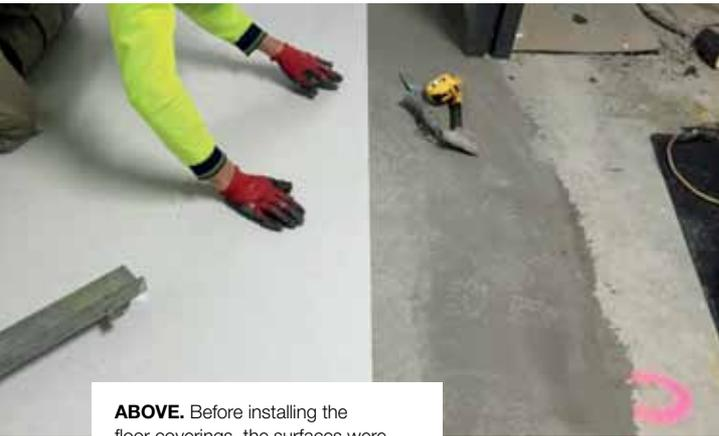
**ABOVE.** Before installing the floor coverings, the surfaces were levelled with ULTRAPLAN. The vinyl floor coverings were installed with ULTRABOND ECO V4 SP.
