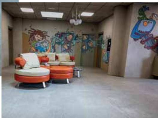
BELOW. Porcelain tiles were installed in the new offices using KERAFLEX MAXI S1 cementitious adhesive. They were then grouted with KERACOLOR GG.
