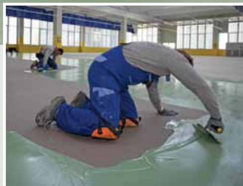
APPLYING Mapefloor I 300 SL BY TROWEL
