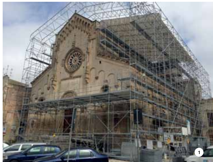
PHOTO 1. The MAPEWOOD system was used for the wooden roof beams and trusses and the MAPEWRAP system was applied to strengthen the structure.
