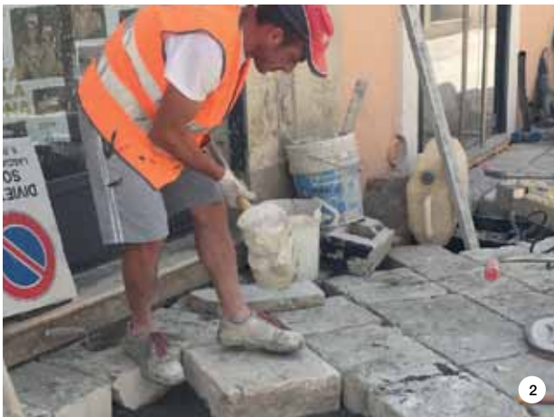
PHOTOS 1 and 2. Installing the paving stones on an installation screed made from MAPESTONE TFB 60.
