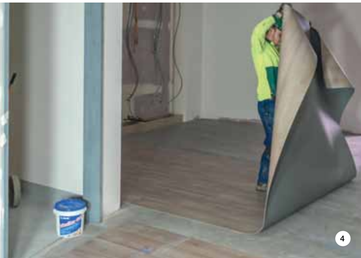
PHOTOS 2 and 3. Some sections of the substrates were repaired with PLANIPREP SC and smoothed with NIVORAPID before bonding the vinyl floors. PHOTO 4. In the bathrooms wall and floor substrates were waterproofed with MAPEGUM WPS. Vinyl floors were then installed with ADESILEX G19. PHOTO 5. In the public areas vinyl coverings were bonded with ULTRABOND VS90 PLUS onto floors and with ROLLCOLL onto walls.
