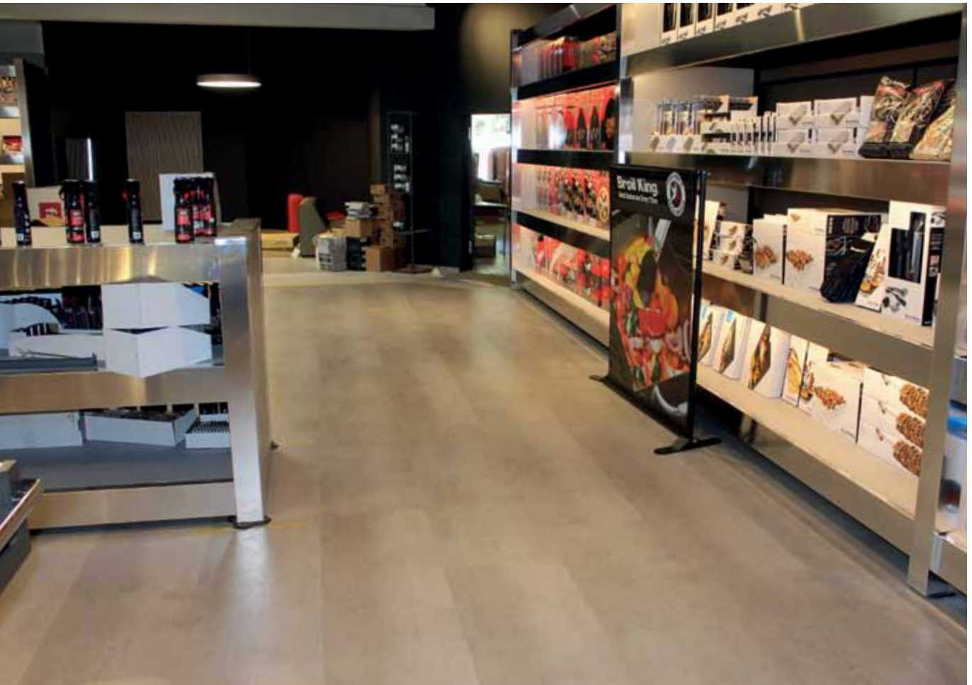
ABOVE. The new LVT floors, properly installed with Mapei products, add a touch of elegance to the shop premises.
