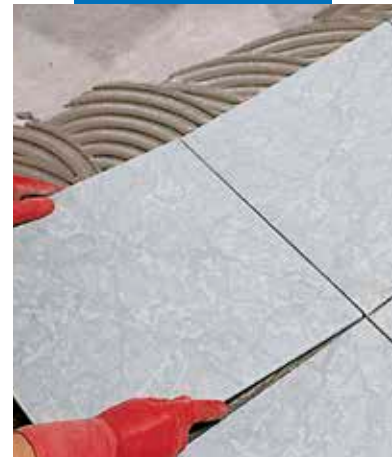
Laying porcelain tiles
