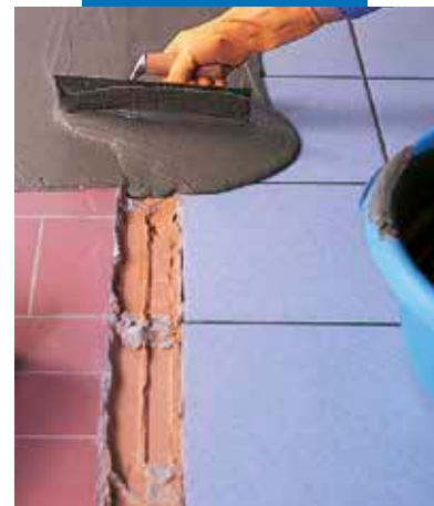
Smoothing existing flooring with Adesilex P4
