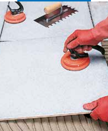
Laying large size tiles
