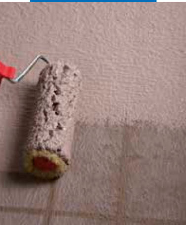
Waterproofing of details by roller
