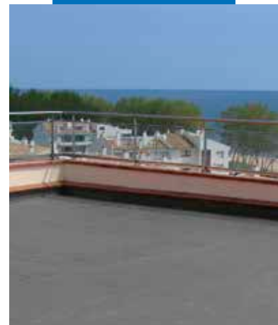
Paving slab waterproofed with Aquaflex Roof
