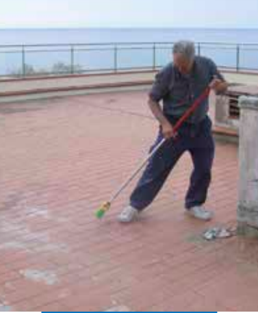
Cleaning a substrate before applying Aquaflex Roof
