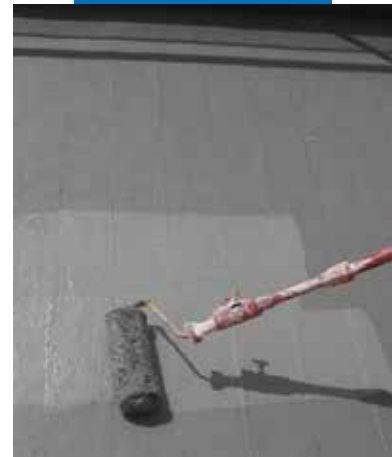
Application of Aquaflex Roof with a long-haired roller
