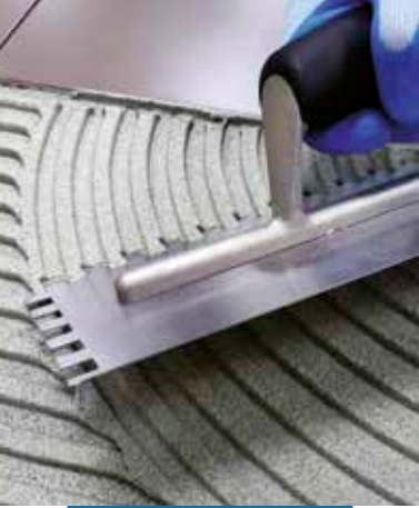
Installation of ceramic tiles in a private residence
