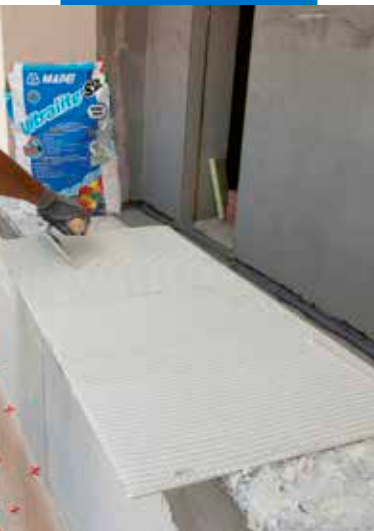
Spreading the adhesive on the back face of the tile
