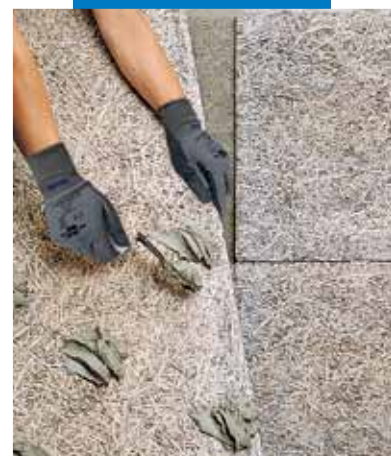
Laying heavy insulation panels
