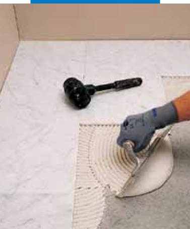
Setting white Carrara marble with Keraquick white
