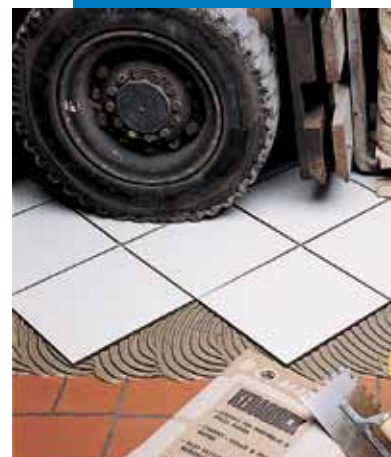
Rapid overlaying on asphalt industrial floor
