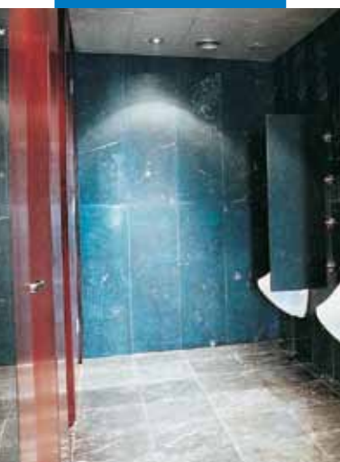
An example of the installation of marble to walls with Keraquick - Feuchtwangen casinò bathroom (Germany)
