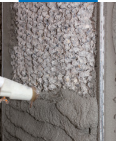
Application of Mapegrout 430 by spray
