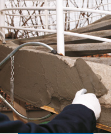
Application of Mapegrout 430 by trowel
