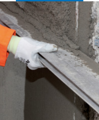
Levelling off Mapegrout 430 with a straight edge
