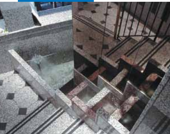
An example of an installation of a granite floor and wall with Keraquick + Latex Plus - Caesaris Palace in Merseyside - Liverpool (GB)
