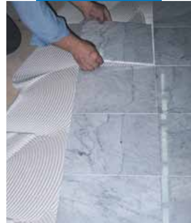
Installing Carrara marble on wooden substrate with White Keralastic
