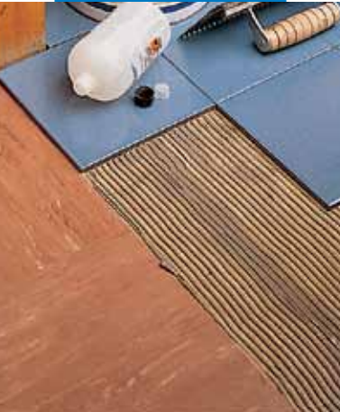
Laying on an old PVC floor
