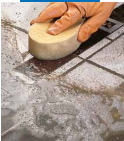
Finishing a ceramic tile floor with wood inlays with a sponge
