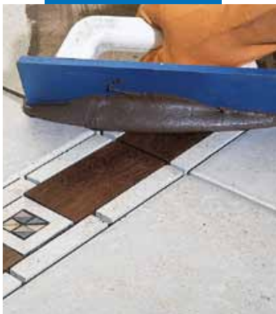
Grouting a ceramic tile floor with wood inlays with a trowel
