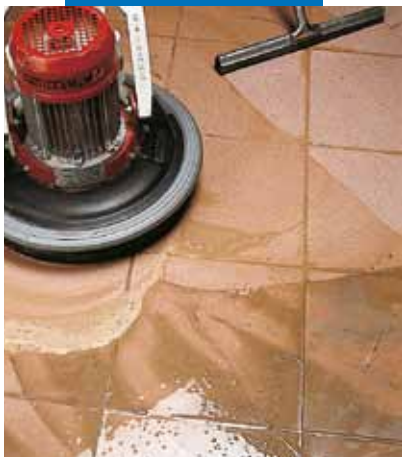
Finishing a porcelain tiled floor with single-brushed power float or rubber squeegee
