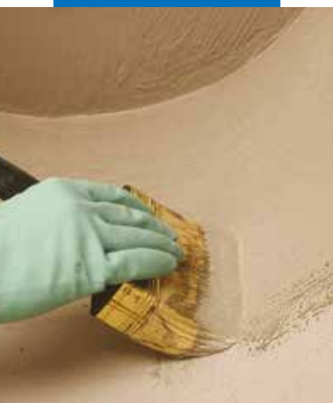
Waterproofing of details by brush
