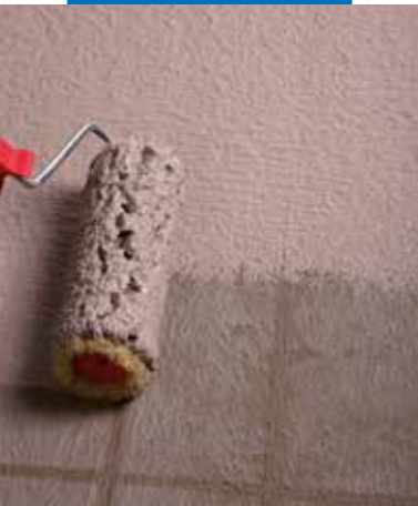
Waterproofing of details by roller
