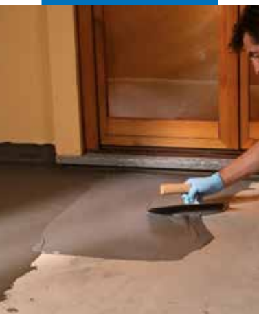
Waterproofing of terraces by trowel
