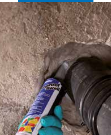
Through element sealed using Mapeproof Swell
