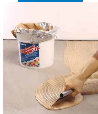
Spreading the adhesive
