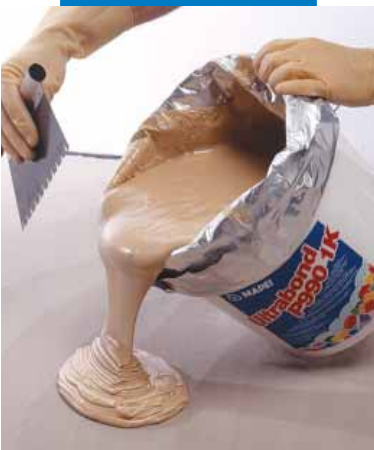
Pouring the adhesive on a screed
