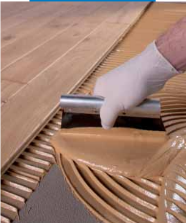
Spreading Ultrabond P990 1K
