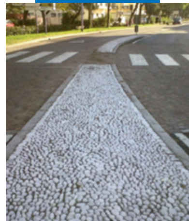
An example of a road with a central reservation in cobblestones
