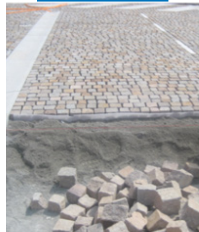
An example of an expansion joint
