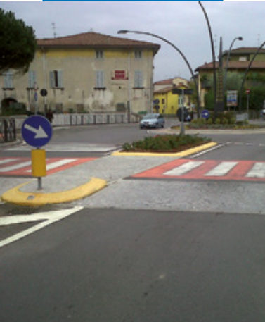
An example of a road hump at a pedestrian crossing
