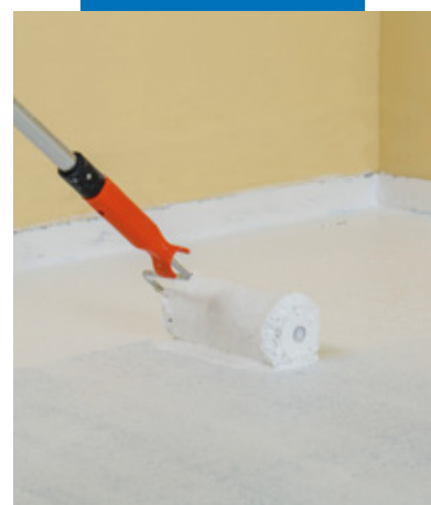
Application of the second coat of Aquaflex Roof Premium
