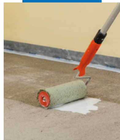
Cementitious substrate primed with Mapecoat I 600 W
