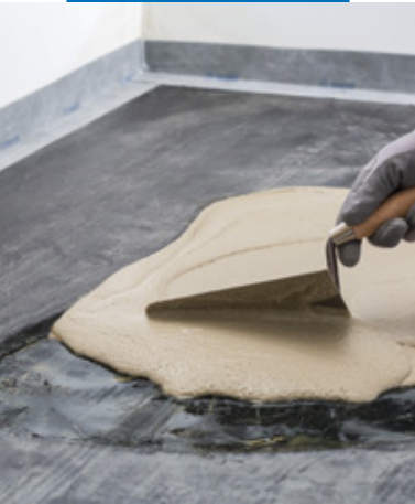
Filling hollows with MapeSlope before applying Primer P3
