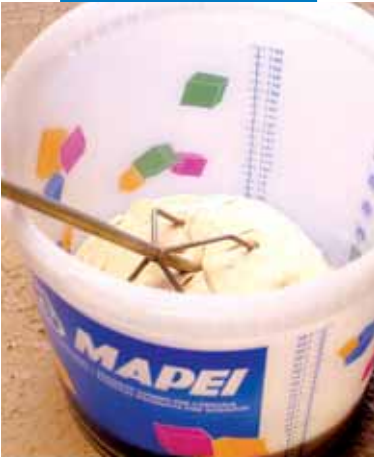
Mapeset mix made with mechanical stirrer
