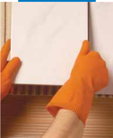
Installation of ceramic tiles on a wall
