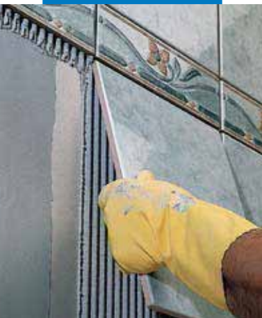
Installation of single-fired tile on wall render
