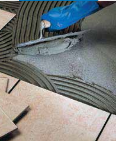
Installation of single-fired tile on floor
