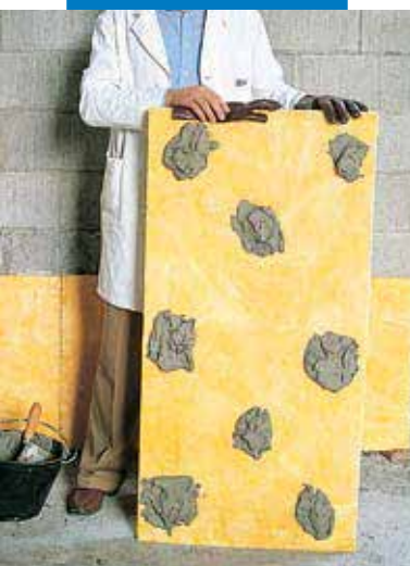
Spot-bonding insulating panels on untreated wall
