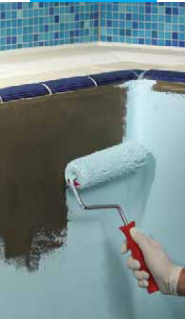
Nanošenje Elastocolor-a Waterproof valjkom
