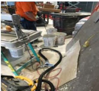
Photo 1. Employee mixing LFT Thinset
