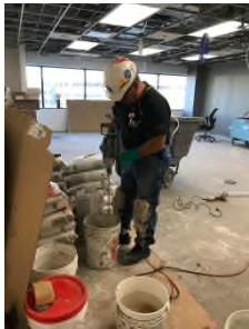
Photo 4. Employee mixing Quickpatch
