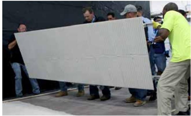
Example of a gauged porcelain tile panel/slab with full mortar coverage
