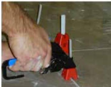
Example of a gauged tile being installed using a mechanical edge-leveling system to reduce lippage
