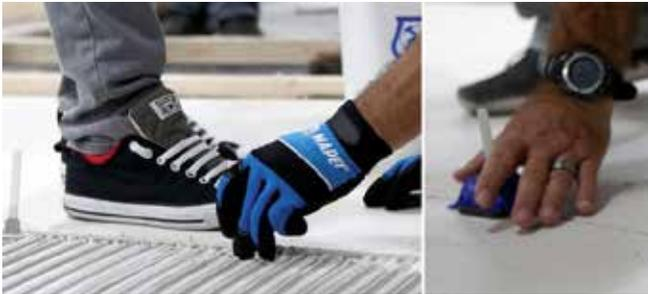
Example of gauged tile over existing tile during a renovation using a mechanical edge-leveling system
