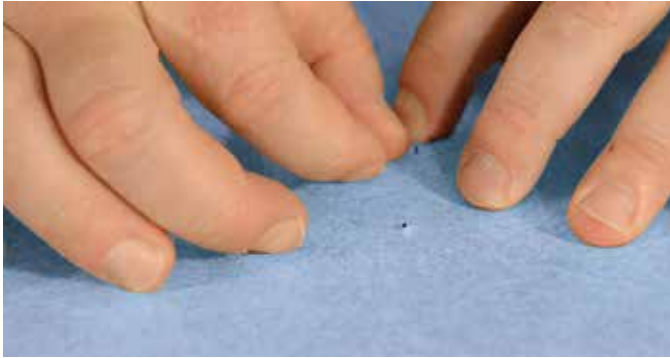
Figure 10: Position Mapelastic WSM over locator pins of the Linear Drain Body.
