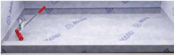
Figure 11: Use a vinyl floor roller to remove any creases or bubbles in Mapelastic WSM .
