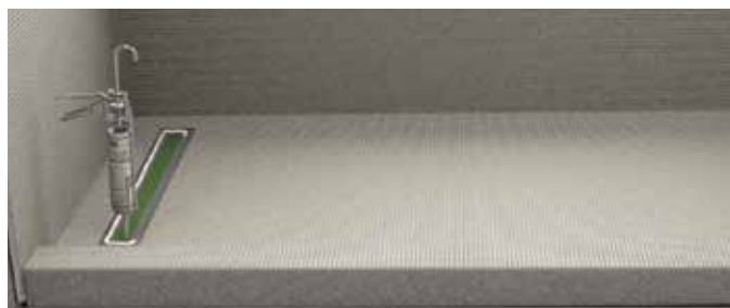
Figure 9: Apply a single bead of ShowerPerfect Hybrid Sealant to the perimeter of the Linear Drain Body.
