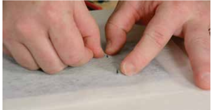
Figure 14: Position Reinforcing Fabric over locator pins of the Linear Drain Body.
