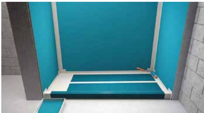
**Figure 12:** Application of *Reinforcing Fabric* and *ShowerPerfect LM Inside Corners* with MAPEI's *Mapelastc AquaDefense*
