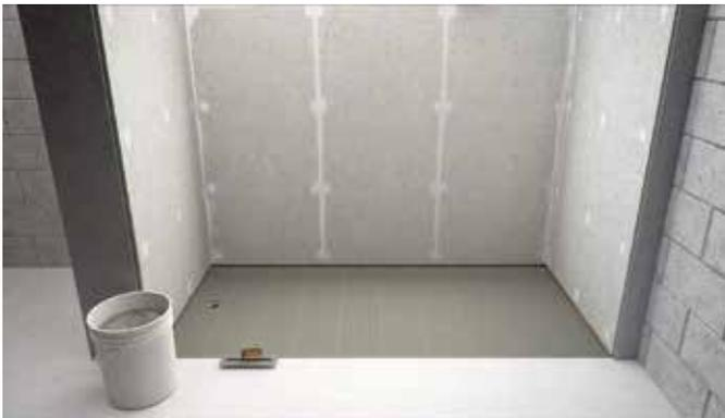
**Figure 6:** MAPEI's *Ultraflex RS* being used to set *ShowerPerfect* pre-sloped pan and drain support frame
