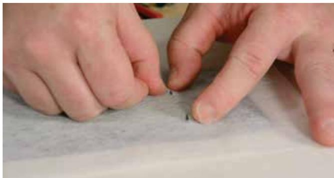
**Figure 11:** Position *Reinforcing Fabric* over locator pins of the Linear Drain Body.
