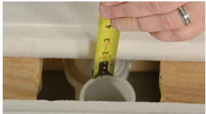
**Figure 5:** Measure from the recessed groove to the top of the "stub-out."
