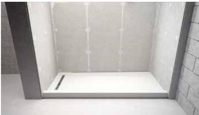
**Figure 7:** *ShowerPerfect* pre-sloped pans and drain support frame installed and ready for next step
