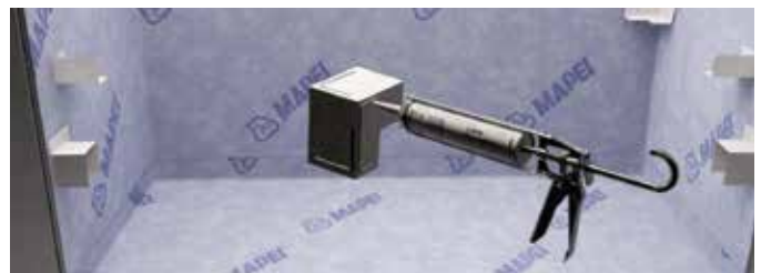
Figure 14: Adhere the pre-formed corners, U-shaped curb cover and 2" (5 cm) overlaps using ShowerPerfect Hybrid Sealant.
