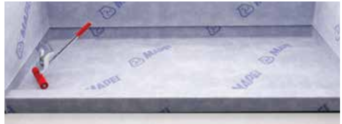
Figure 13: Use a vinyl floor roller to remove any creases or bubbles in Mapelastic WSM .
