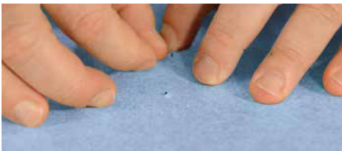
Figure 12: Position Mapelastic WSM over locator pins of the Linear Drain Body.
