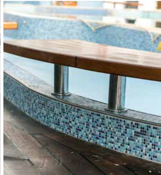
LEFT: Crews applied Mapecoat Guard 100 as a primer, followed by Mapedeck Litescreed polyurethane underlayment mixed with Marine Filler 20 . CENTER: MAPEI's marine-certified line is new to the U.S., but has been very successful in Italy. RIGHT: When installing tiles and pool mosaics, the crew used Kerapoxy as a mortar and Kerapoxy CQ as a grout.
