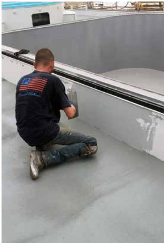
LEFT: Crews applied Mapecoat Guard 100 as a primer, followed by Mapedeck Litescreed polyurethane underlayment mixed with Marine Filler 20 . CENTER: MAPEI's marine-certified line is new to the U.S., but has been very successful in Italy. RIGHT: When installing tiles and pool mosaics, the crew used Kerapoxy as a mortar and Kerapoxy CQ as a grout.
