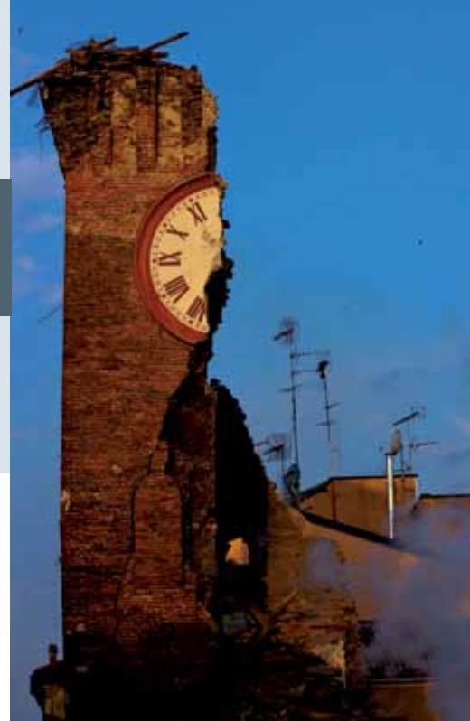
Rubble after the earthquake in 2012: the remains of the bell-tower of the church in Correggioli (Ostiglia).
