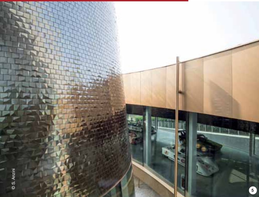
PHOTO 5. The substrates of the cones were waterproofed with PURTOP 1000. The 3D ceramic tiles were installed with ULTRABOND ECO PU 2K and the joints were grouted with ULTRACOLOR PLUS.
