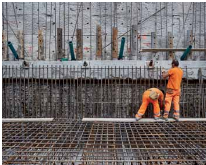
ABOVE. An overall view of the area where the work was carried out. IN THE FACING PAGE. Excavation and construction work to widen the section of the bed of the Bisagno Stream. BELOW. Preparation work carried out before pouring the reinforced concrete for the new structures.
