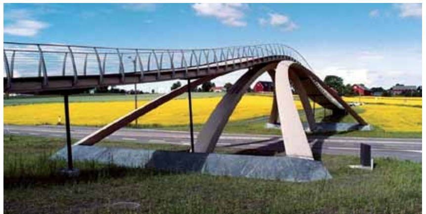
The Da Vinci bridge was built in Ås, in Norway, by using a design by Leonardo Da Vinci.
