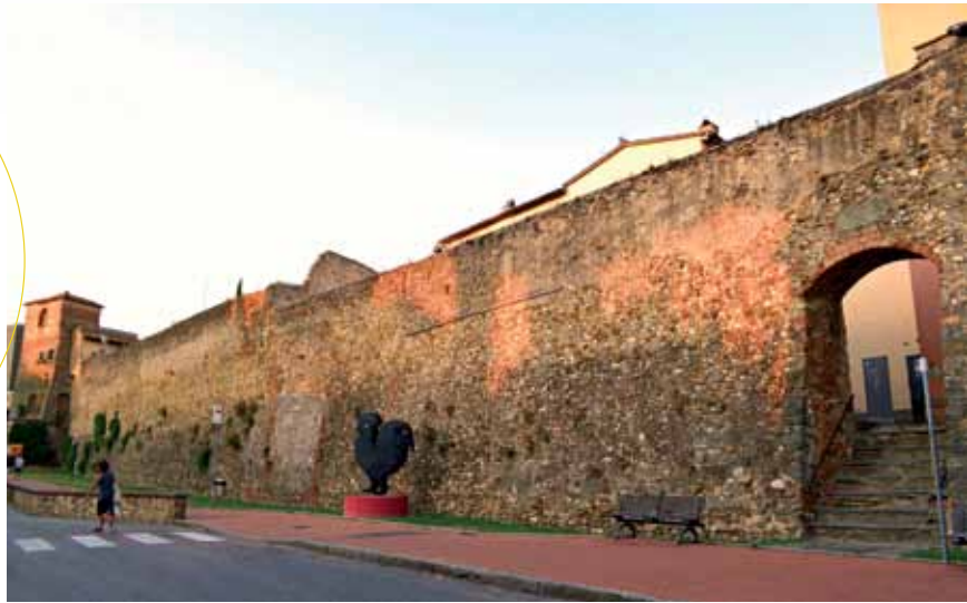
Florence city walls were renovated by using Mapei solutions for masonry repair.
