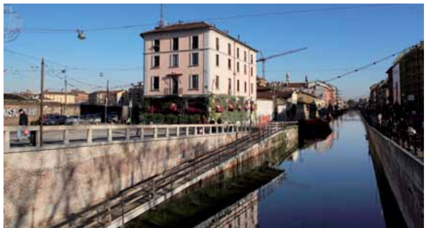
Mapei took part in the conservative restoration of the Naviglio Grande Canal in Milan.
