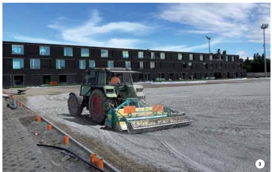
Spreading and mixing MAPESOIL 100
