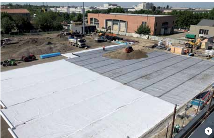
View from above: positioning the geofabric and geomesh
