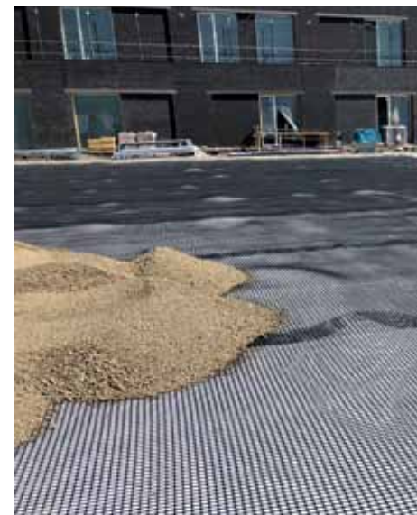
Applying the road base material
