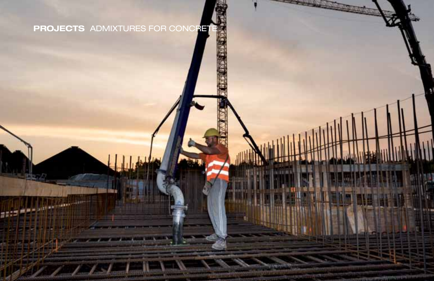
33,000 m 3 of concrete were pumped non-stop for 94 hours last May to build the foundation slab of the hospital.
