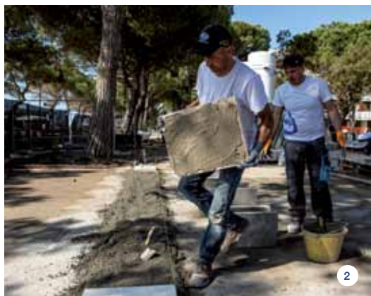
PHOTO 1. Applying the bonding slurry prepared with PLANICRETE on the rear side of a stone slab.
