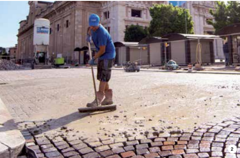
1. Installation of the paving with MAPESTONE TFB 60. 2. Grouting the joints with MAPESTONE PFS2 FLEX.
