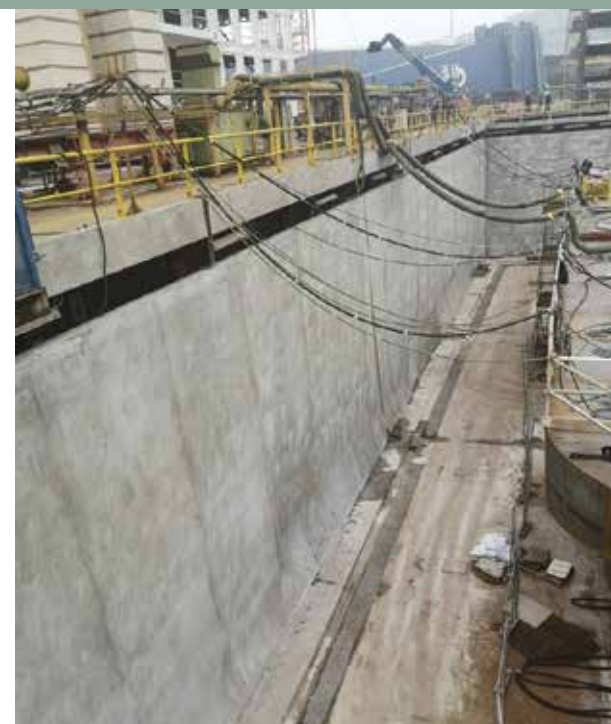
IN THE FACING PAGE. A view of the Fincantieri shipyard in Marghera, near Venice. ABOVE. Reinforcing rods were protected with MAPEFER anti-corrosion mortar (left), while several Mapei solutions were used to waterproof and repair the dock walls (right).
