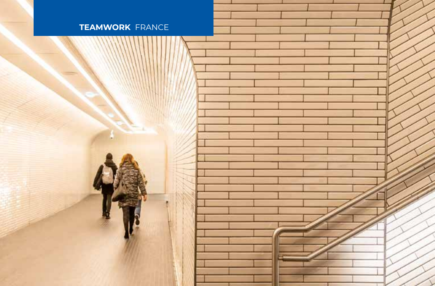
Ceramic floor and wall tiles were installed in the new stations along Line 14 using Mapei products such as GRANIRAPID, KERALASTIC T, ULTRALITE S2 QUICK and ULTRACOLOR PLUS.
