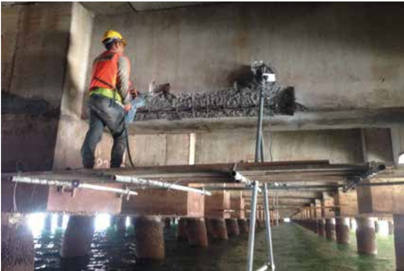
ABOVE. Kuantan Port is a multipurpose port in the East Coast region of Peninsular Malaysia. LEFT. Damaged concrete areas were removed and reinforcement rods were protected with MAPECOAT ZR MY, fast-drying, zinc-rich coating. Underwater concrete elements were repaired with MAPEFILL MC 06.
