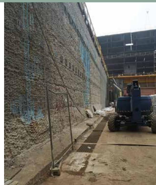
IN THE FACING PAGE. A view of the Fincantieri shipyard in Marghera, near Venice. ABOVE. Reinforcing rods were protected with MAPEFER anti-corrosion mortar (left), while several Mapei solutions were used to waterproof and repair the dock walls (right).
