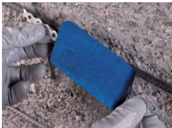
MAPESHIELD anodes are connected to the reinforcement rods so that the zinc they are made of oxidises over time, protecting the reinforcement.
