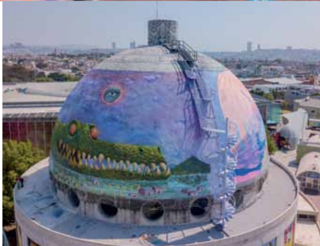
MANUEL GÓMEZ MORÍN CULTURAL CENTRE. In Queretaro, the Cúpula del Péndulo de Foucault, a 2,000 m 2 dome overlooking the library of this Cultural Centre, was waterproofed with AQUAFLEX TECHOS FIBRADO*. The cupola was then painted with murals by local and international artists.
