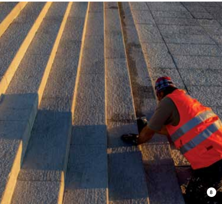
PHOTO 8 . Skirting was bonded in place with KERAQUICK MAXI S1.
