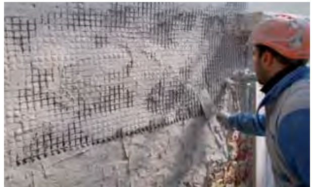
Application of a compact strengthening layer to increase the shear and tensile strength of masonry walls using the FRCM System.
