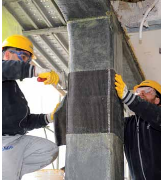
Strengthening a beam-pillar junction with MAPEWRAP C SYSTEM.
