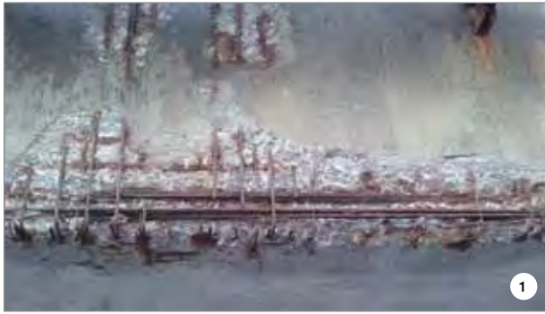
PHOTO 1. An example of a reinforced concrete damaged by corrosion of the reinforcement rods.
