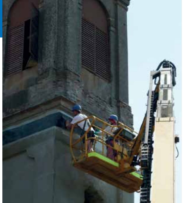
The Church of Camposanto (Italy), damaged by the earthquake, was renovated using Mapei systems for structural strengthening.
