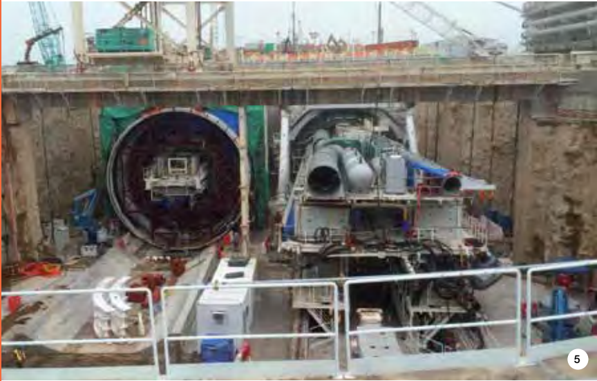
PHOTO 5. The largest tunnel boring machine in the world while boring the subsea tunnel section.
