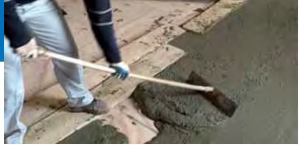
Strengthening a wooden floor using PLANITOP HPC FLOOR.
