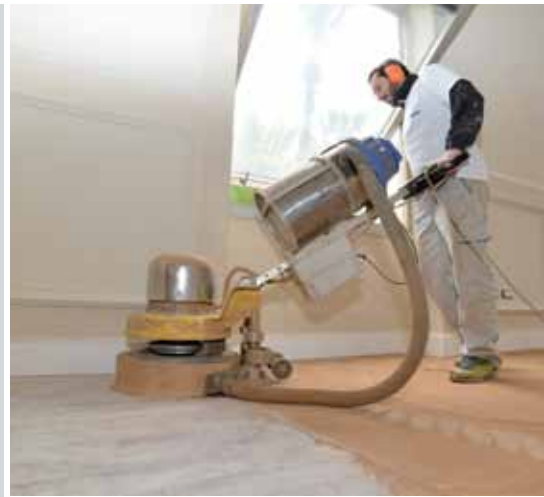
The substrates were sanded around one hour after applying ULTRACOAT BINDER, which is mixed with sawdust. The surfaces were then finished with ULTRACOAT HIGH TRAFFIC varnish.
