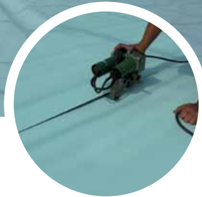
The water tanks were waterproofed using MAPEPLAN T WT.
