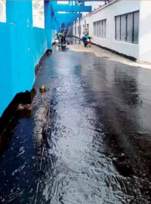
LEFT. The floors in the corridors and on the stage were waterproofed with PLASTIMUL PU membrane. RIGHT. PLANISEAL 288 mortar was applied to waterproof the substrates in the bathrooms and showers.
