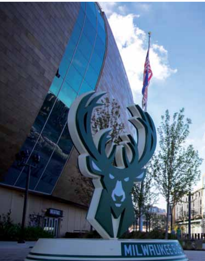
An exterior view of the Fiserv Forum.
