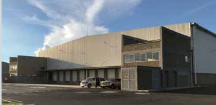
LEFT. The Mapei Colombia plant in Bogotá.
