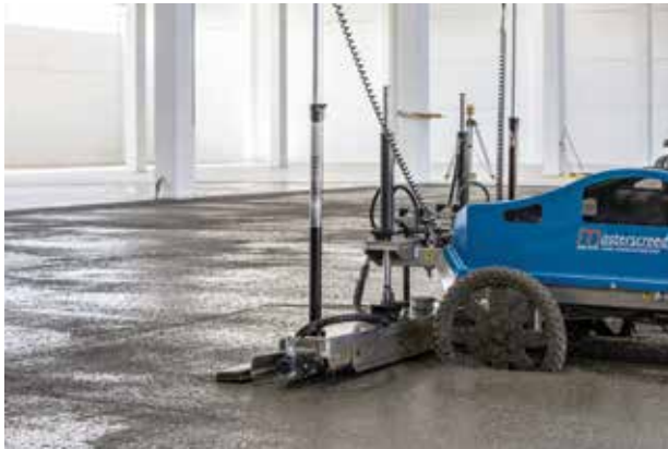
ABOVE. Some of the installation phases of the floor: left, offloading concrete; right, placing the concrete with a laser screed machine
